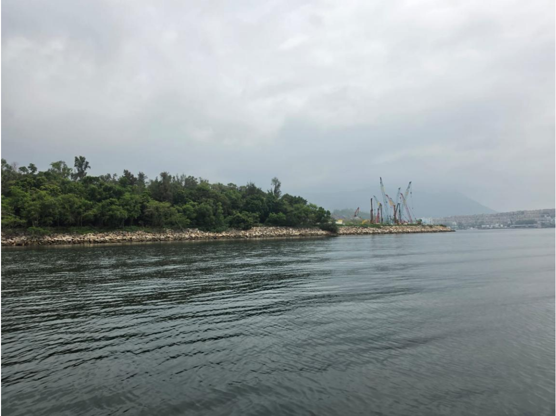
Photos taken by the Environmental Team on 20/05/2026
